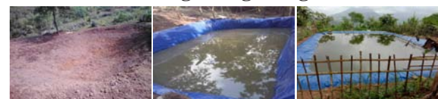
Fig 16b. Construction of Jalkund at Hukphang village
