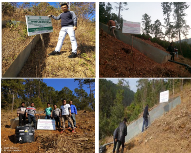
Fig 18. Installed runoff structure under various slope gradients and fallow jhum period
