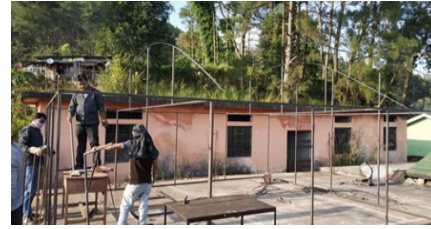
Fig 23. Construction of frame for Solar smart tunnel dryer
