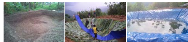
Fig 16a. Construction of Jalkund at Mongtikang village
